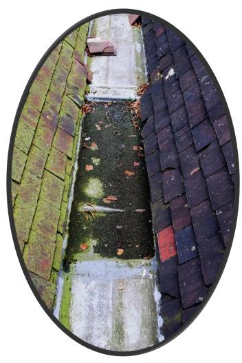
Broken pieces of tile slide down the roof into the leadlined valleys and puncture the lead sheet. Over the years there have been many repairs to the leadwork, but the time has come to replace many tiles, the lead and the wooden underboarding that supports it.
