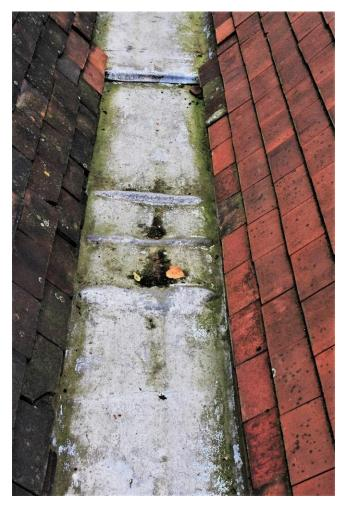
During the last hundred and fifty years the lead has moved with changes of temperature, creating folds in the lead; the folds develop cracks allowing water ingress. The Victorian practice was to use long lengths of lead sheet; unfortunately, with changes of temperature this causes a lot of movement due to expansion and contraction.
